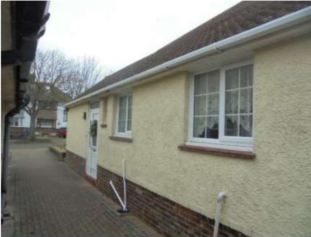
Side elevation - facing Millcross Road, Millscross Rd to left
