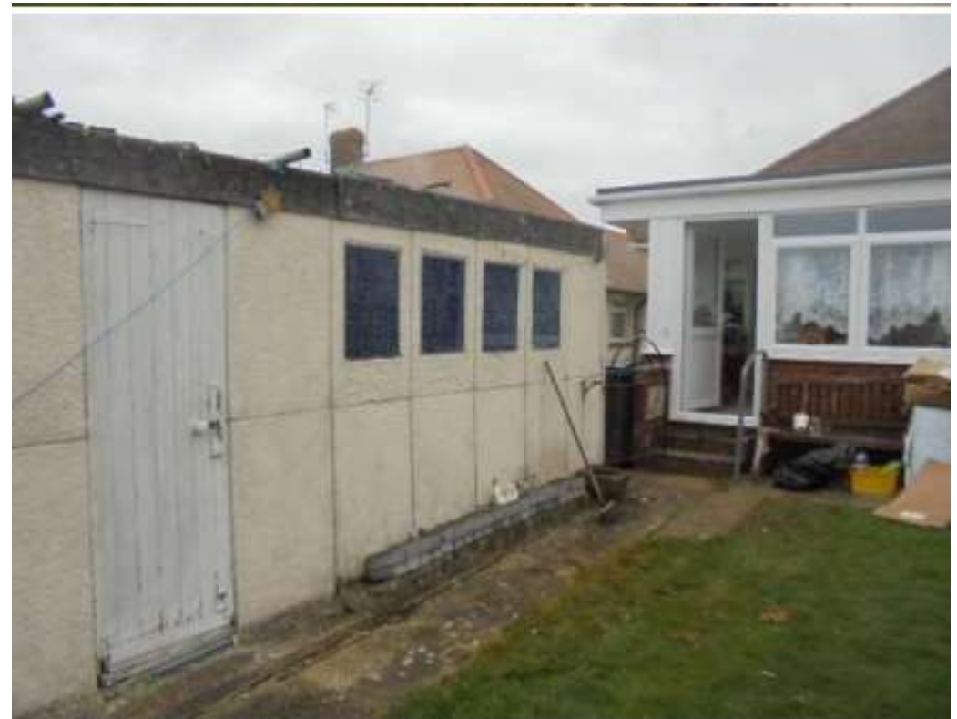
Outbuilding along western site boundary – facing north
